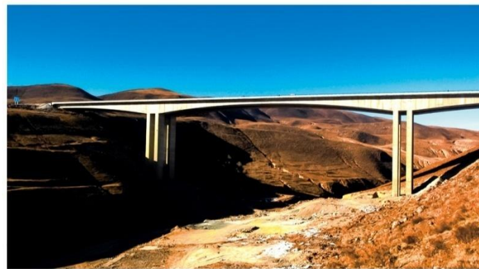
内蒙古集丰高速公路 Jining - Fengzhen Expressway Project in Inner Mongolia
