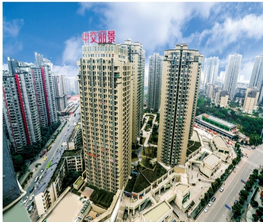
重庆中交丽景七号地块三标段工程 Lot 3 Project of Chongqing CCCC Lijing No. 7 Plot
