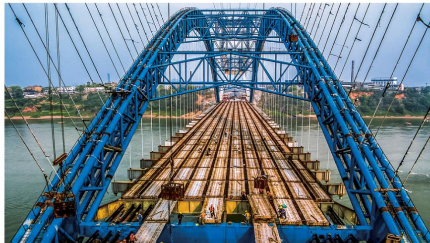
湖南湘潭市湘江四大桥 Fourth Bridge over Xiangjiang River in Xiangtan, Hunan
